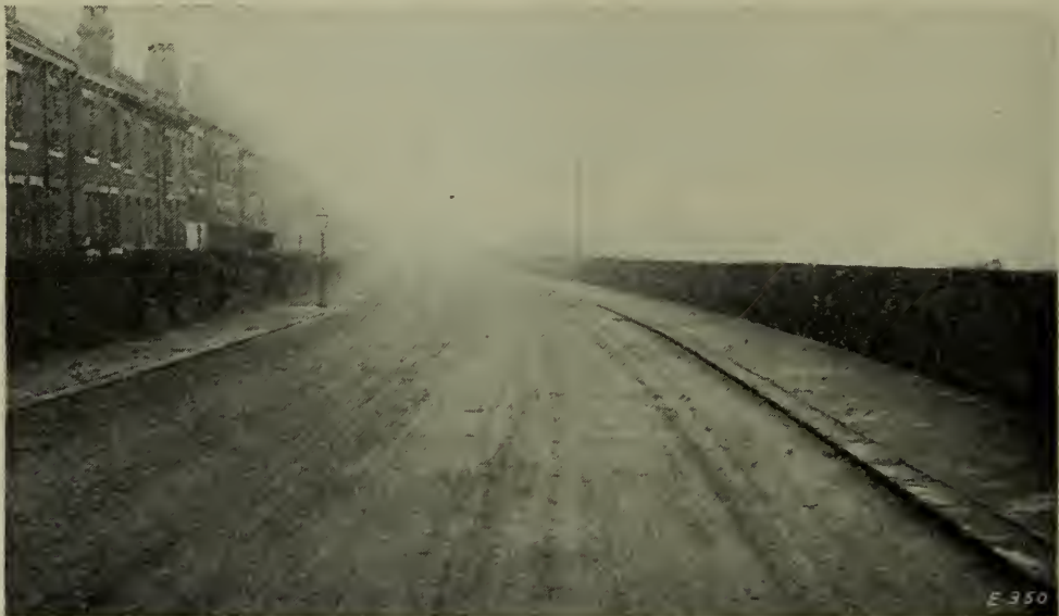
GARNET ROAD, SIX MONTHS AFTER COMPLETION.
